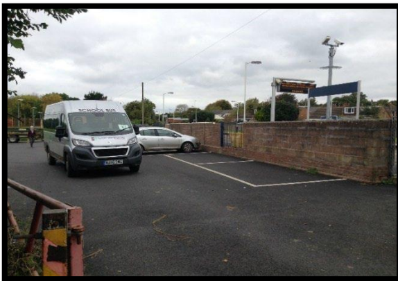
Pinhoe Station Car Park
