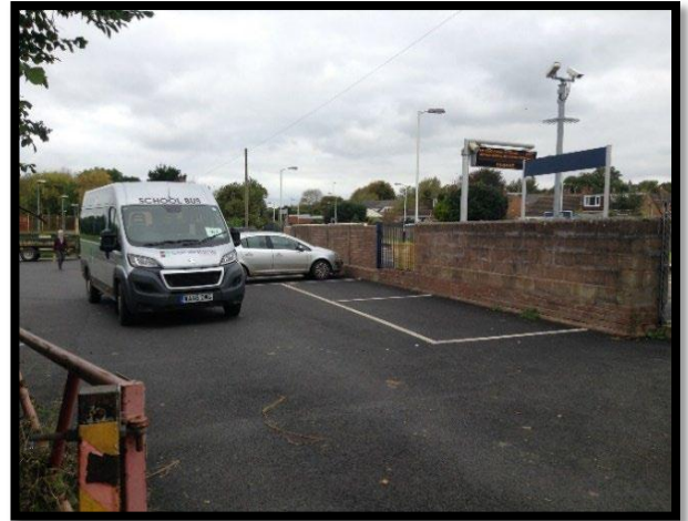
Pinhoe Station Car Park
